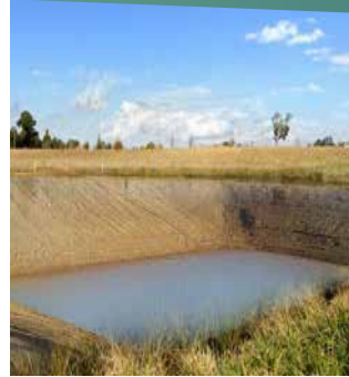
Before using Aquatic Dam Stop Leak Professional
