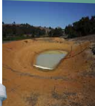
Leaking dam walls
