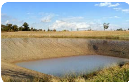
Before using Aquatic Dam Stop Leak Professional
